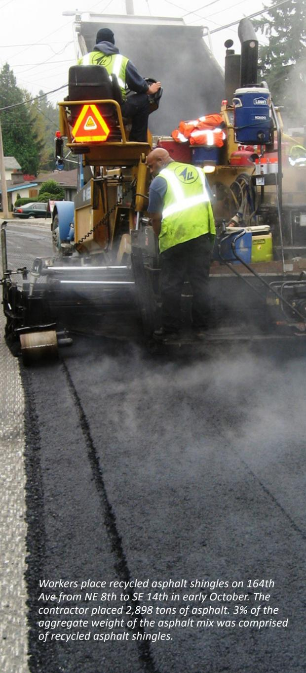
Workers place recycled asphalt shingles on 164th Ave from NE 8th to SE 14th in early October. The contractor placed 2,898 tons of asphalt. 3% of the aggregate weight of the asphalt mix was comprised of recycled asphalt shingles.
